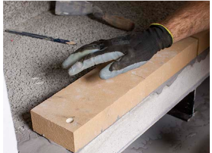
Bed the firebricks on to a 3mm layer of firebrick mortar. Use the tables on the previous page as a guide.
