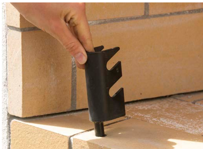
Drill 2 x 12mm diameter holes in the front row of the firebricks. Push log retainer holders in place.
