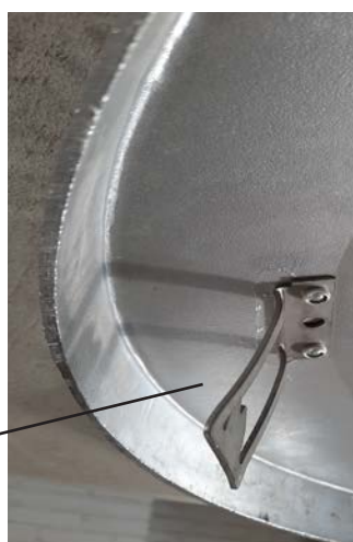
Bend the steel prongs out so the top ring is a tight push fit into the concrete capping.
