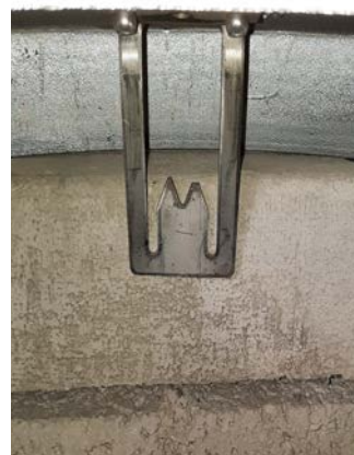
Bend the steel prongs out so the top ring is a tight push fit into the concrete capping.
