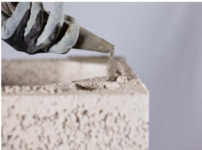
If extra chimney blocks are purchased, simply repeat the adhesive steps to add them on top of the previous block.
