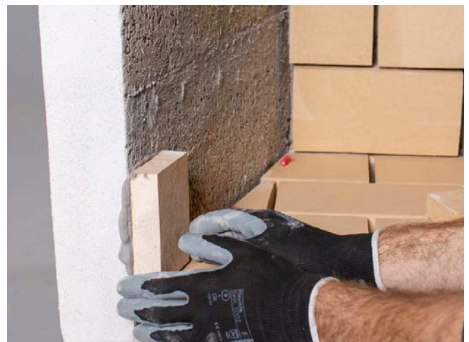
Once the bottom and rear firebricks are in place, fasten the side bricks in position using the firebrick mortar. Use a tile spacer to keep an 8mm gap. During the first and second level, you must slot in the grill supports as shown in the next step →
