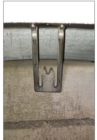
Bend the steel prongs out so the top ring is a tight push fit into the concrete capping.
