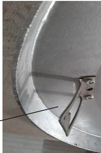
Bend the steel prongs out so the top ring is a tight push fit into the concrete capping.
