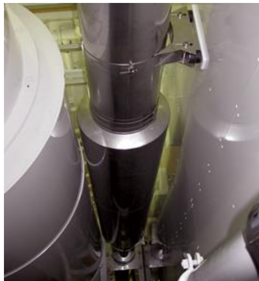
Metaloterm® resonance silencers are divided into two noise reduction levels on average are between 20 and 30 dB.
