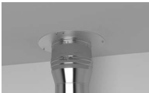
2-piece fire stop plate attached securely to joists
