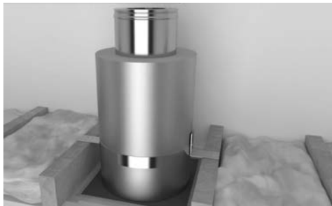
Protect Box lowered into position and fastened securely to the joists
