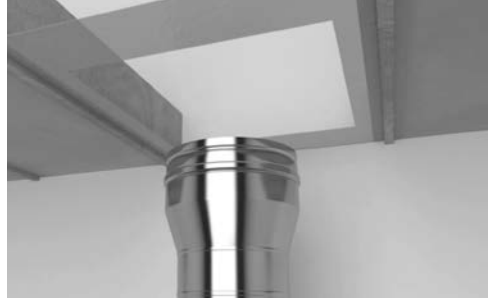
Square section cut out of barrier
