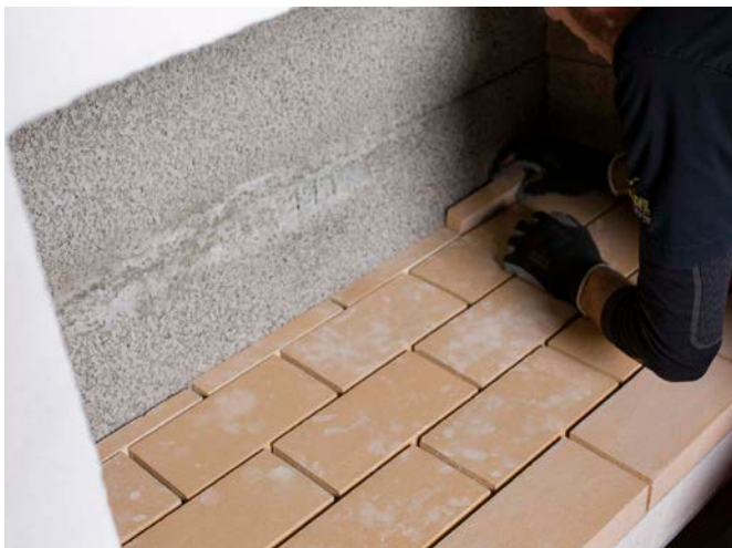
Complete the bottom layer of firebricks, then fasten the rear firebricks in place using the firebrick mortar. Use a tile spacer to keep an 8mm gap.
