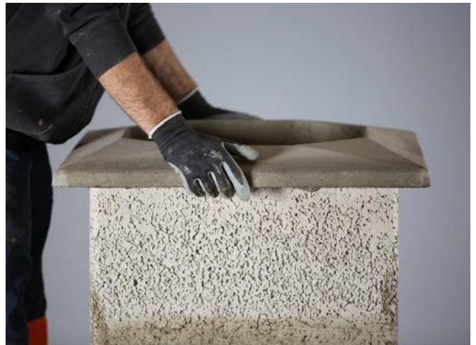
Glue on the capping.
